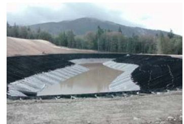
South Pond during Construction at Issaquah Highlands
