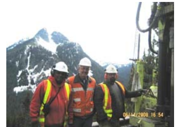
Chinook Pass Roadway Washout Drilling to Evaluate Repair Options
