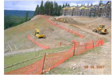
Suncadia Resort's Bullfrog Pit Restoration during Lodge Construction
