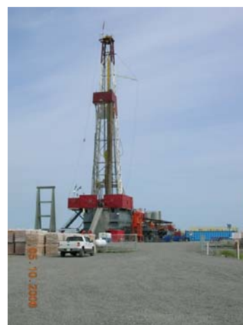
Drilling Anderville Farms #1 Natural Gas Exploration Well
