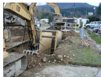
Regional Water Facility Extension during Construction
