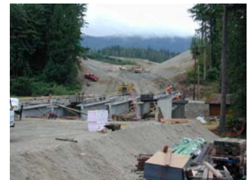
North SPAR during Construction – North Fork Issaquah Creek Bridge
